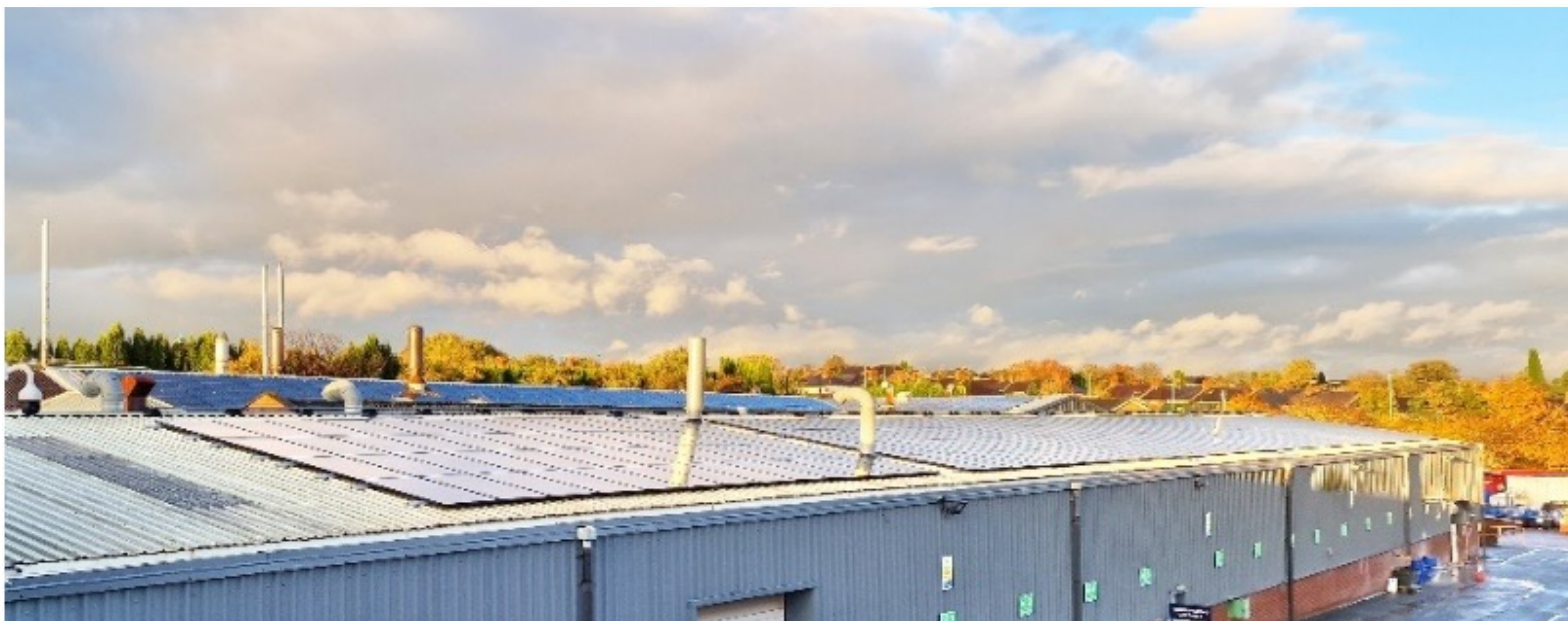
Credit: Churchill China - Solar Panel installation
